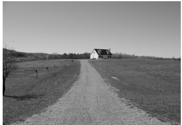
3B. The access to this house traverses the middle of an open field and cuts directly across contours, becoming the dominant feature in the view and adversely impacting the visual appeal of the open field.
