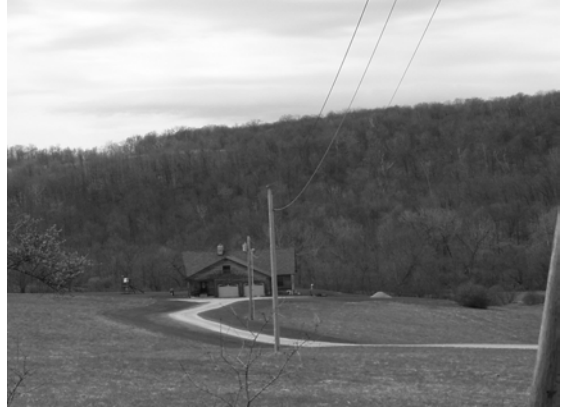
2B. Above-ground utility lines cutting across the open field to the house at the back edge detract from the scenic quality of the field.
