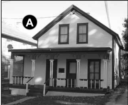
Fig. 5-72: 126 Jefferson St. The strong use of contrast in the paint colors of this building highlight the trim work.
