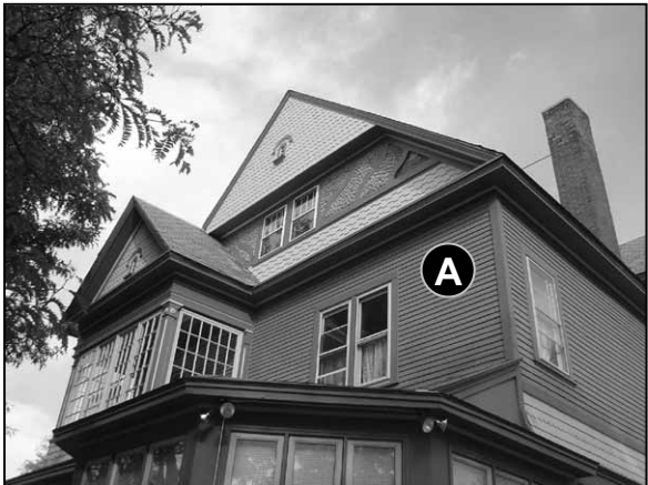
Fig. 5-75: 185 North St. Different paint colors are used consistently to distinguish clapboards, shingles and stonework on this building.
