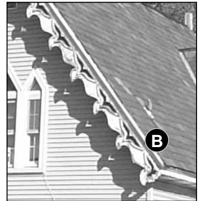
Fig. 5-49: 207 Depot St. The intricate eave on this house defines much of the architectural character, and should be protected.
