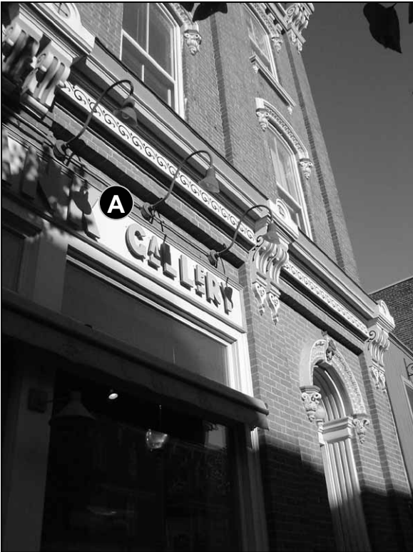
Fig. 5-84: 332 Main St. Applied lettering framed within the design of the façade is often the cleanest solution.
